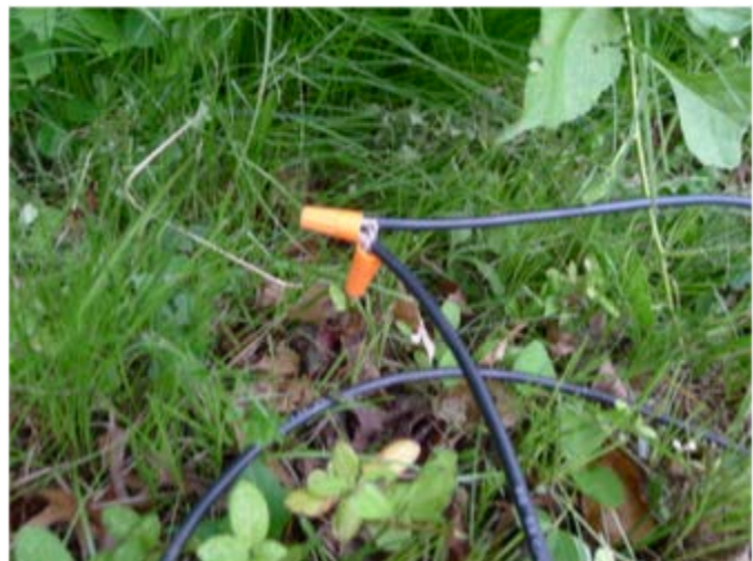
FIG. 5. Repairs are straightforward and can be made weatherproof and permanent if desired.
