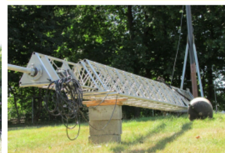
TOWER ALMOST READY TO GO BACK UP
