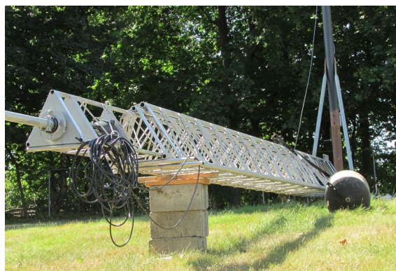
TOWER ALMOST READY TO GO BACK UP
