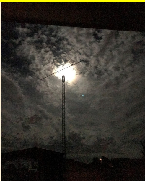
N1API CAUSING SOME CORONA DISCHARGE ON HIS BEAM
