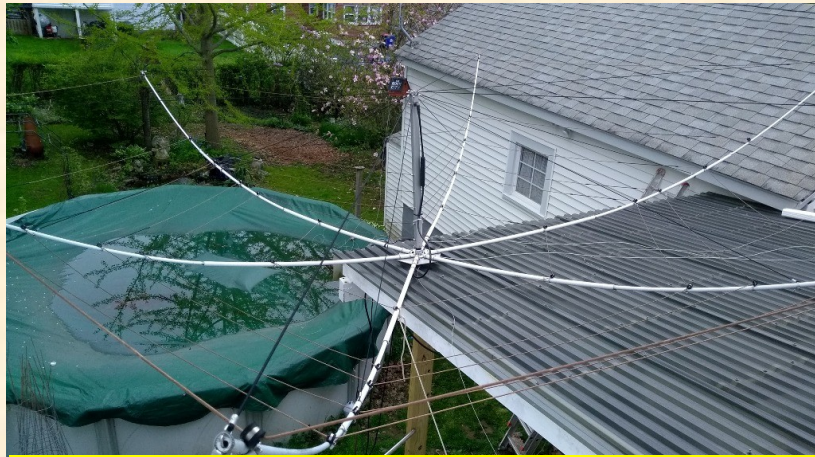
KC1SA SPIDER BEAM WAITING TO GO BACK UP AFTER DECK REPAIRS
